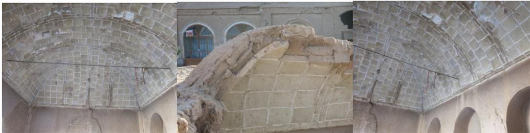
**Figure 1: Samples of interior and exterior images of Kermani vault**
