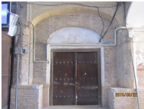
Fig 2- House entrance door
