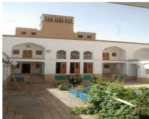
Fig 7- Interior yard-wind tower
